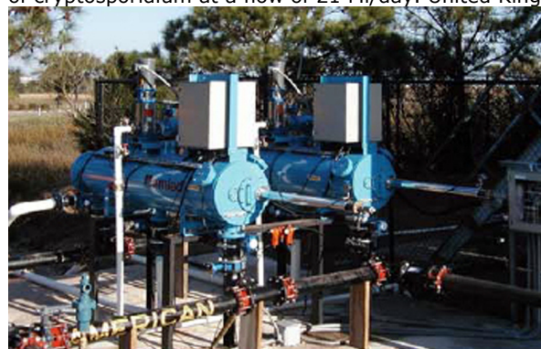
WWTP – Tertiary Discharge Compliance. 60 m 3 /h, 10μ Harbor Island – Beaufort, SC. USA
