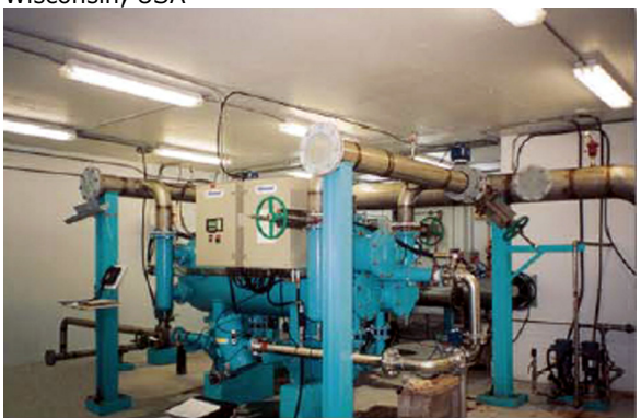
Intake to DWTP, 136 m 3 /h, 3μ to prevent Giardia. Deer Lake, Canada
