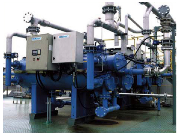
Removal of carbon particles and fine fibers for reuse of wastewater. 170 m 3 /h. Abekawa Paner mill. Japan
