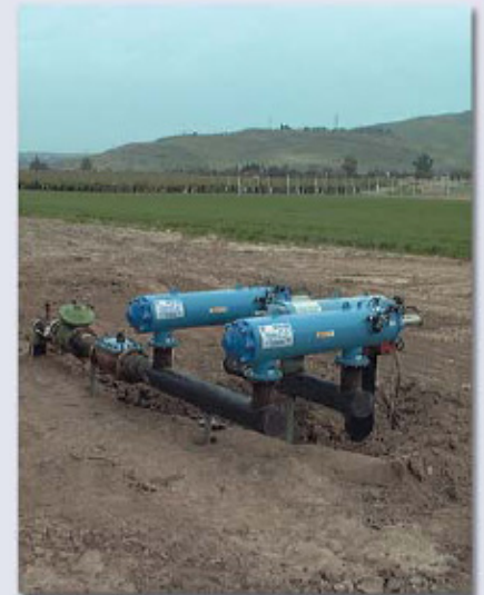
▲ Lake water used for drip irrigation. 130µm. Sea of Galilee, ISRAEL
