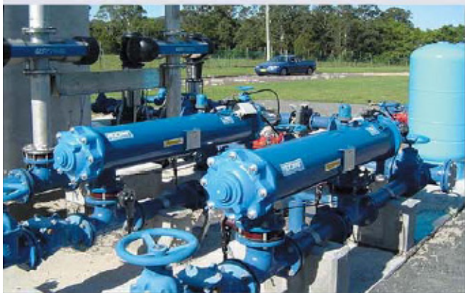
▲ Treated sewage water for irrigation of pasture. 200µm. Stroud Sewage Treatment Plant, Stroud, NSW, AUSTRALIA
