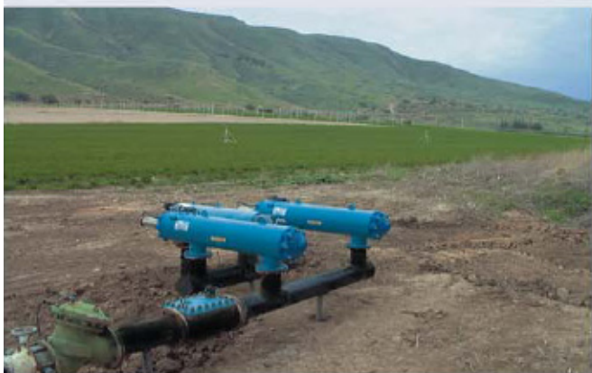
▲ Filtration of well water. Up to 150m³/h, 80µm. Potable water supply system. ISRAEL
