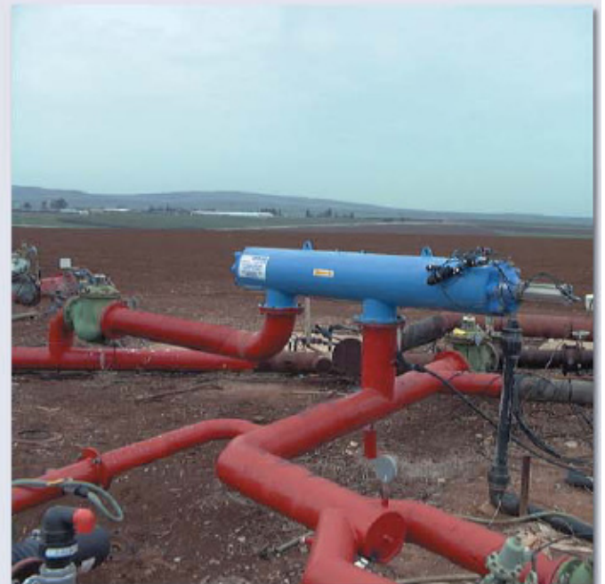
▲ Filtration of reservoir for drip irrigation. 130µm. Israel
