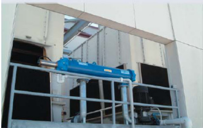
▲ Cooling tower side stream filtration. 100µm. Eastlands Plaza Shopping Centre, Ringwood (Melbourne), AUSTRALIA
