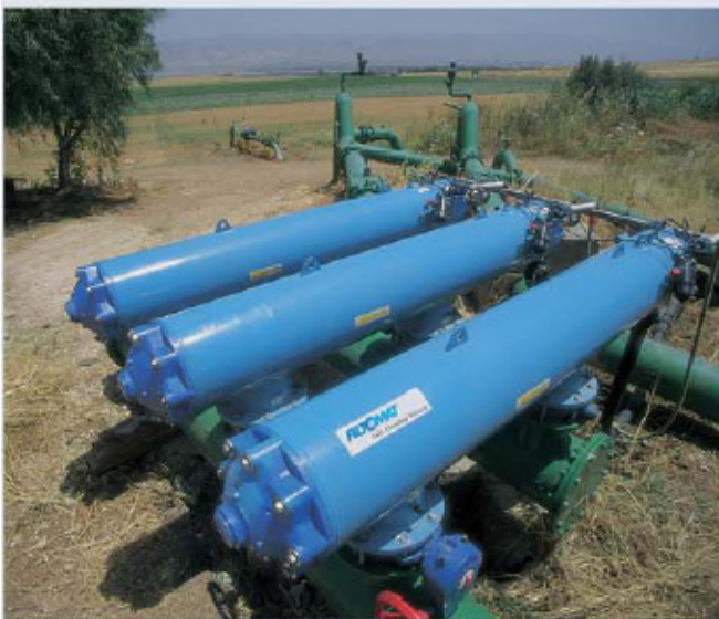
▲ Filtration of flood water for irrigation. 200µm. ISRAEL
