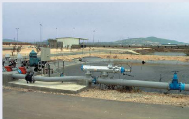
▲ Wastewater reservoir. Pre-filtration to drippers. 400µm. ISRAEL
