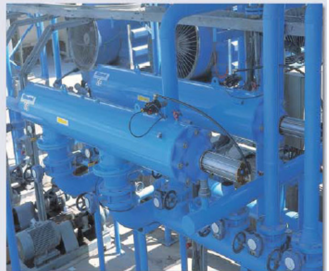
▲ Cooling water filtration. 50µm. Detergents manufacturer. ISRAEL
