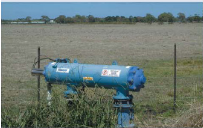
▲ Treated sewage effluent water for landscape irrigation. 200µm. Bunnerong Cemetery, Bangholme (Melbourne), AUSTRALIA
