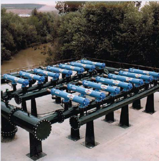
▲ River water filtration for drip irrigation. Palma del Rio, SPAIN
