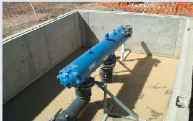
▲ Treated sewage effluent water for landscape irrigation. 130µm. Sandhurst Estate, Carrum Downs (Melbourne), AUSTRALIA
