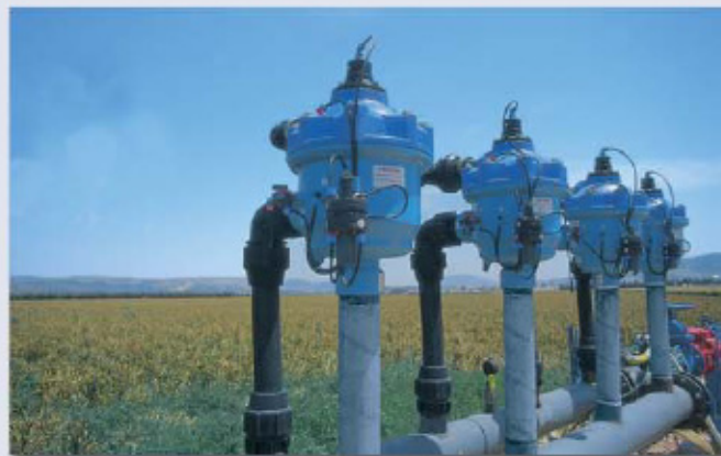
▲ Drip irrigation of row crops. 120m³/h, 130µm. Afula, ISRAEL
